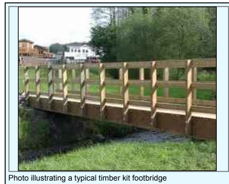
Photo illustrating a typical timber kit footbridge
