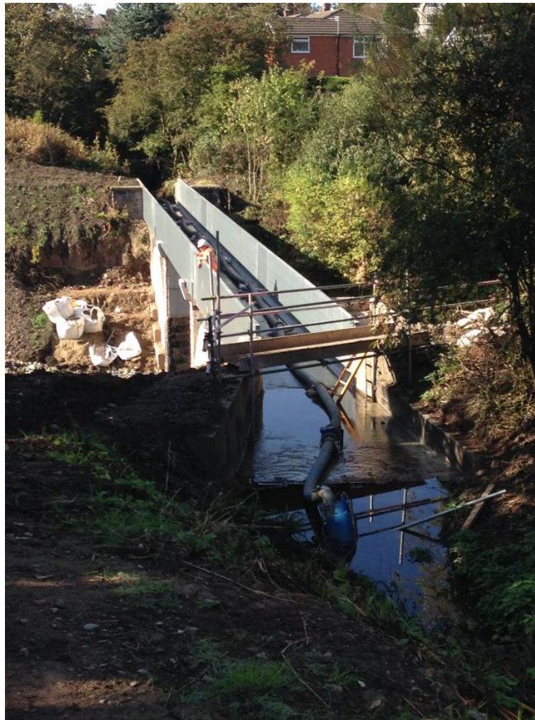
River Chor aqueduct near Chorley
